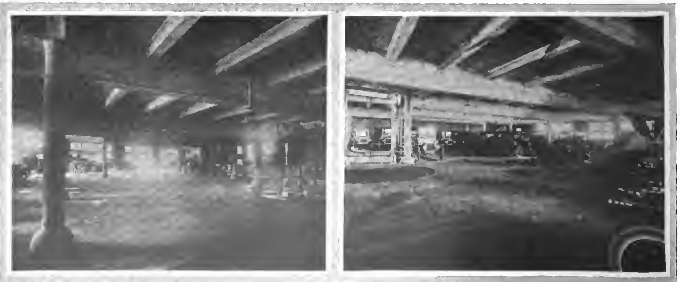
View on Second Floor, Devoted to Live Storage. Also Third Floor, for Dead Storage
